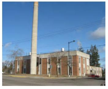
architecting and administering the support systems and server farm for all of Facilities and Planning. The Central Heating and Cooling Plants provide high pressure steam and chilled water to the Utility Tunnel System that basically brings the steam and chilled water to most buildings on the EWU campus. Condensate return is also brought back from the buildings on campus through the utility tunnel system.
